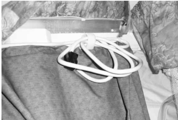
Air Conditioner cord stows at ceiling under curtain with VELCRO. MAKE SURE TO STOW ON TAKE-DOWN BEFORE PUSHING IN BEDS.
